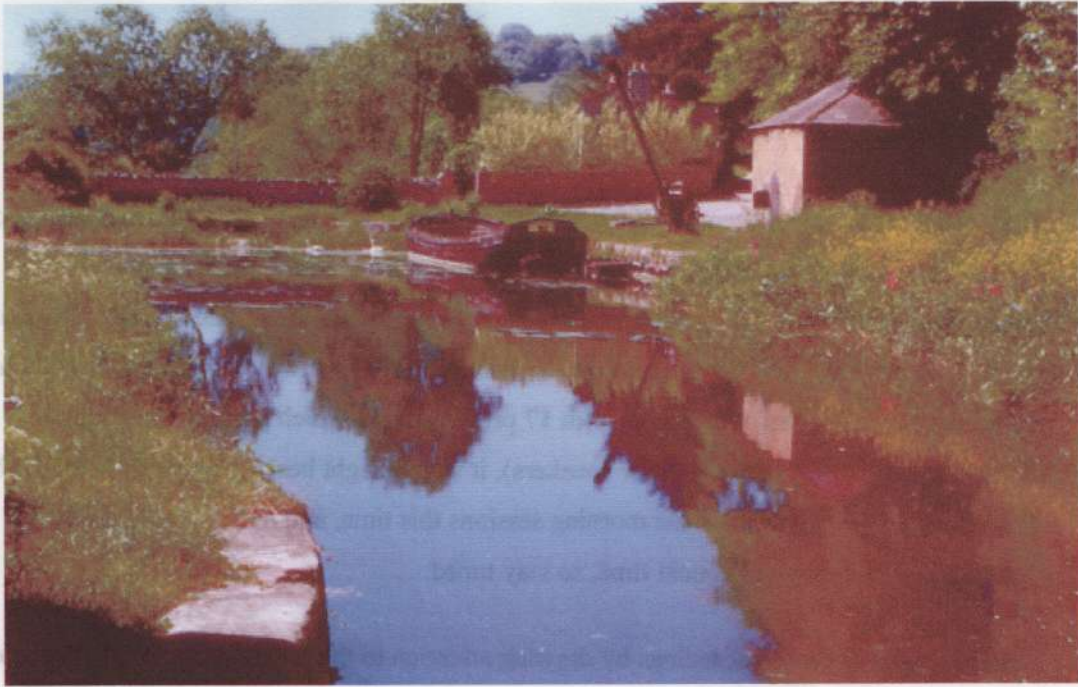
A waterlogged and derelict trow at Dundas Wharf 1962. At this point the Somersetshire Coal canal joined the Kennet and Avon canal.
