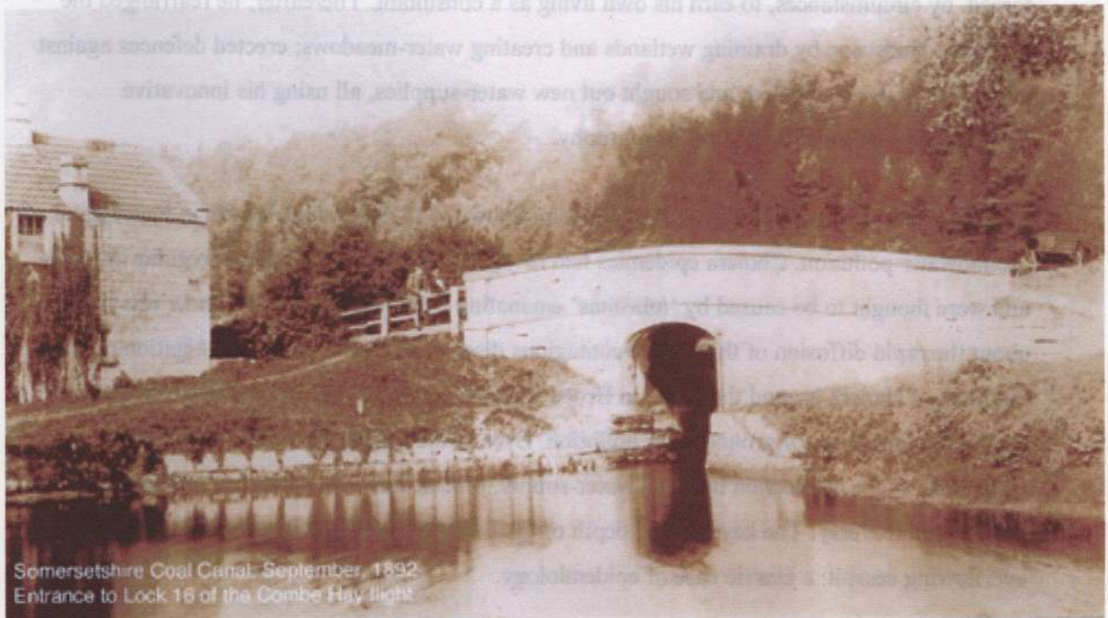
The Somersetshire Coal Canal at Combe Hay, photographed in September 1892. The bridge crosses the entrance to lock 16 in a flight of 22 joining the upper & lower levels of the canal between Midford Wharf and Paulton Wharf.
